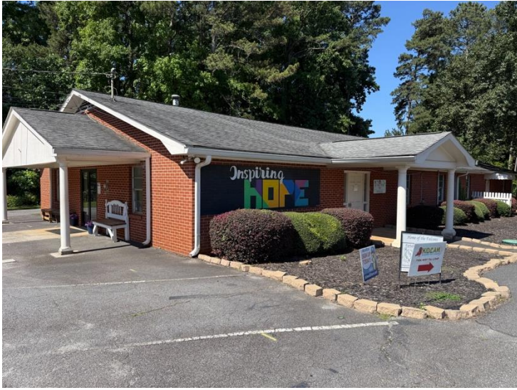
Brick Assembly Building
