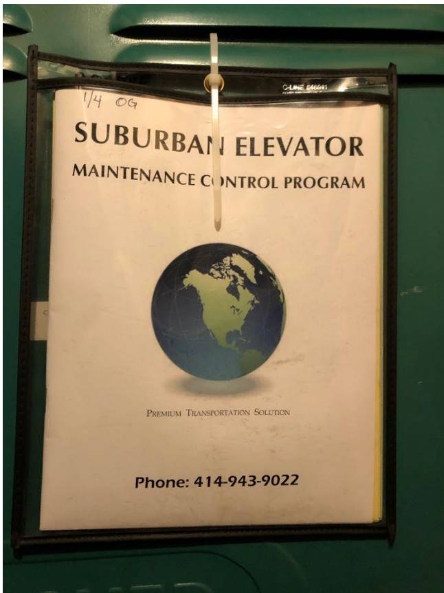
Properly maintained hydraulic elevator
