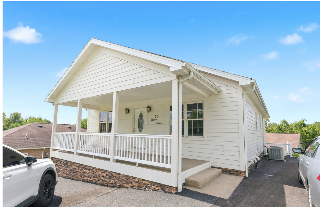
15 Crammeys Run Road (Upper Level).
