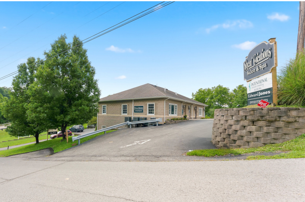
Access to Upper Level 933 Cheat Road, 15 Crammeys Run Road and Garage.
