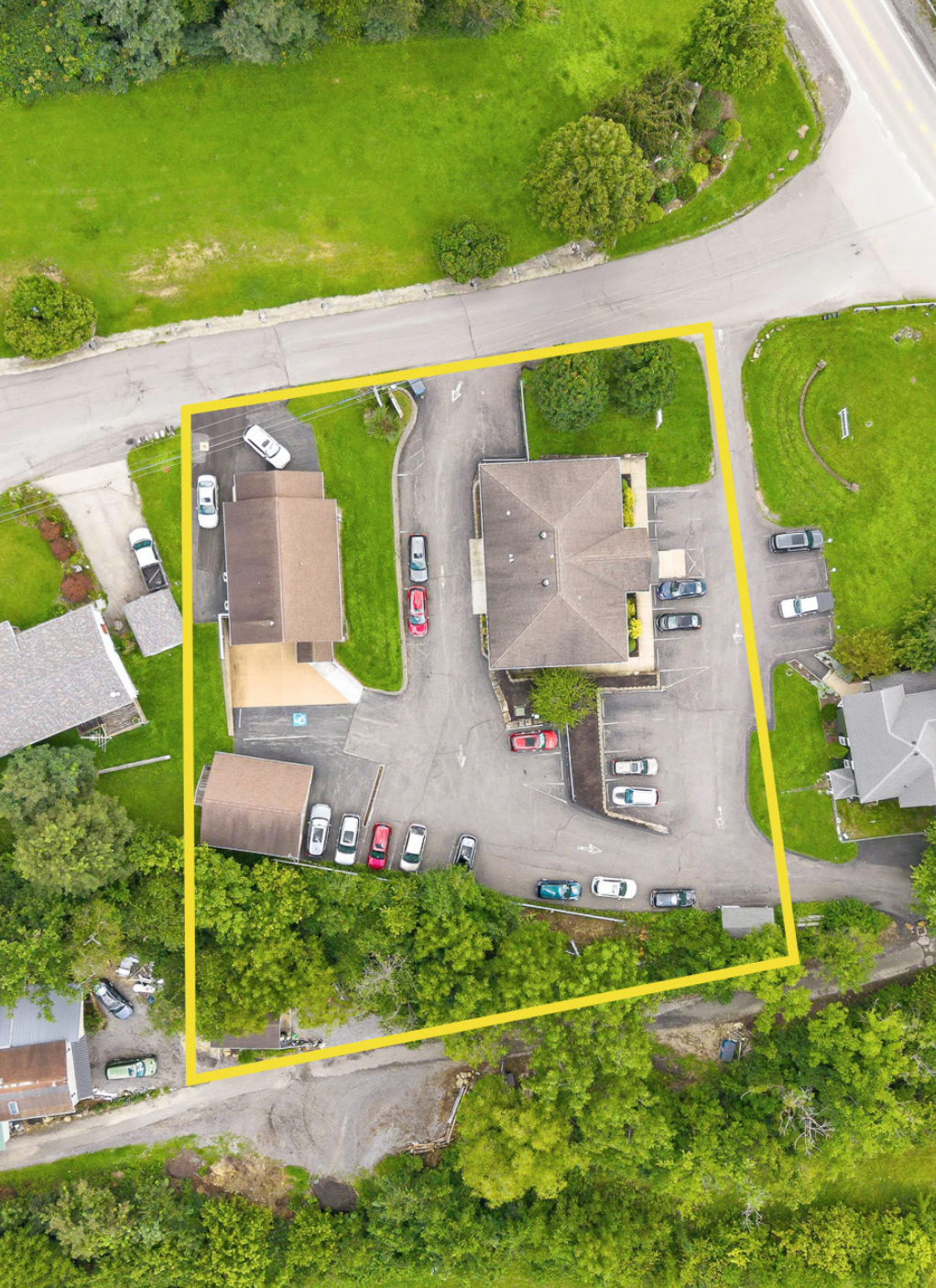
Aerial View From Above.
