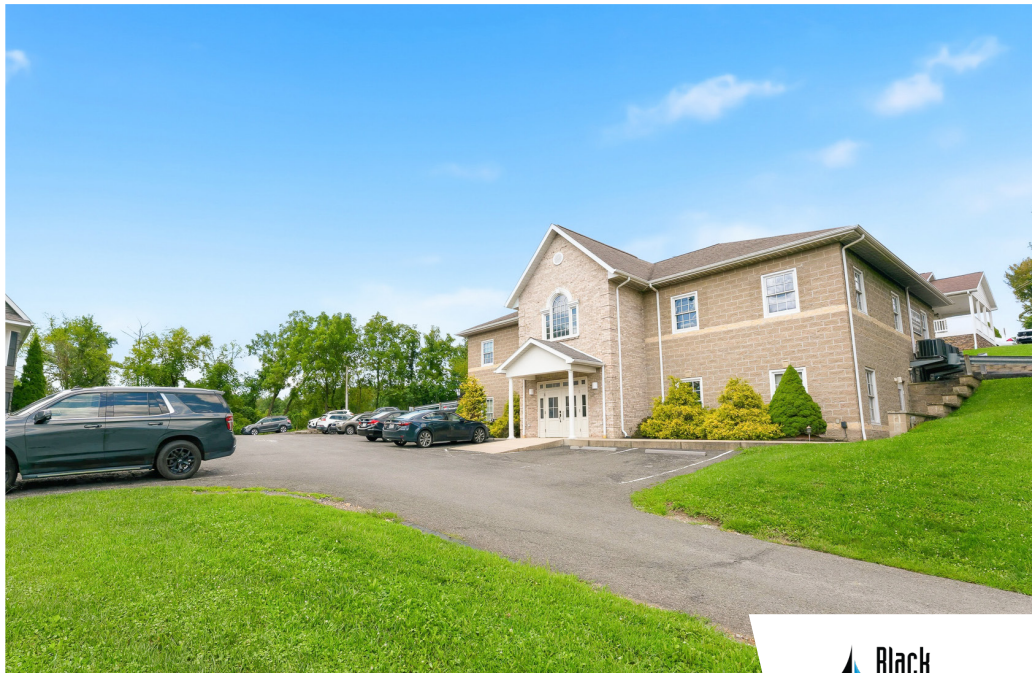
Access to Lower Level 933 Cheat Road.
