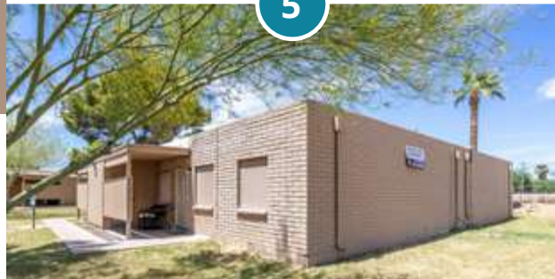
APACHE ROAD APARTMENTS 180 N. APACHE ROAD | BUCKEYE
