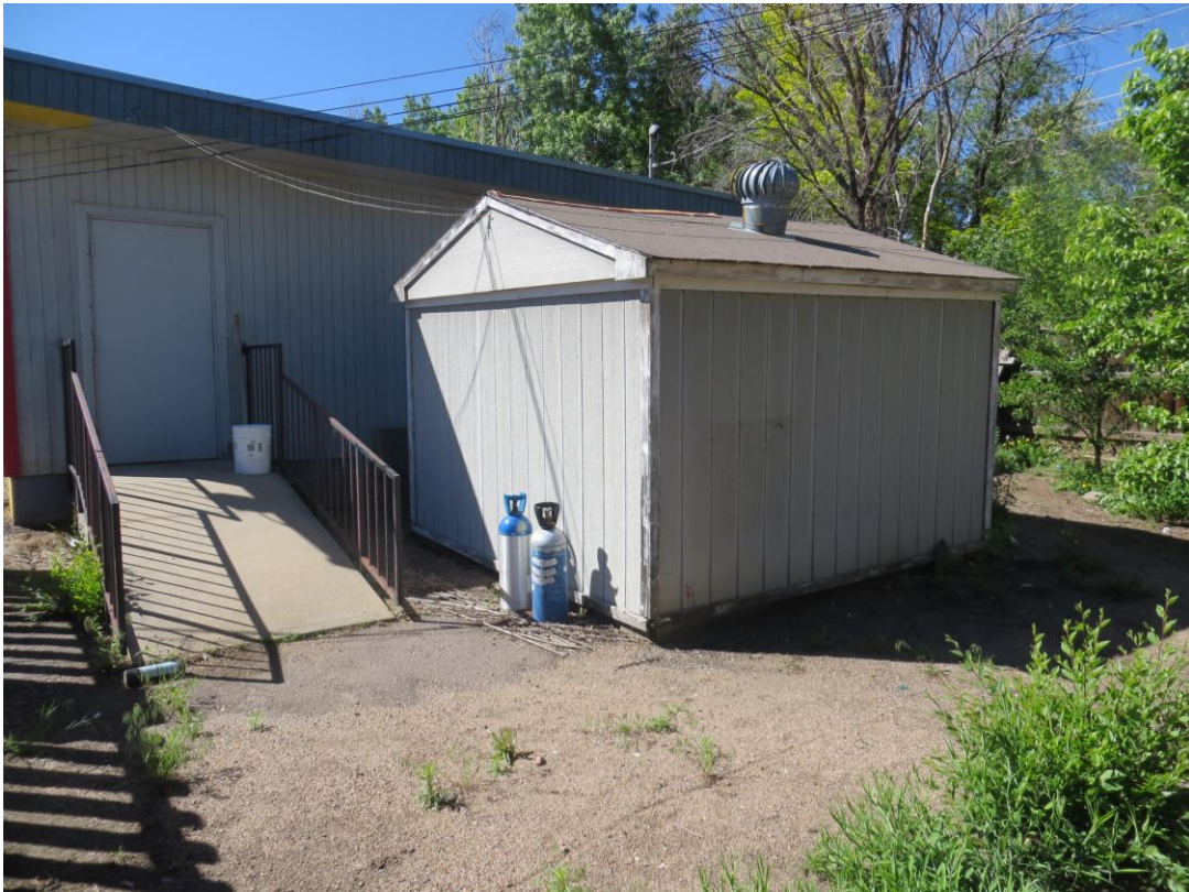
A storage shed at the northwest end of the building.
