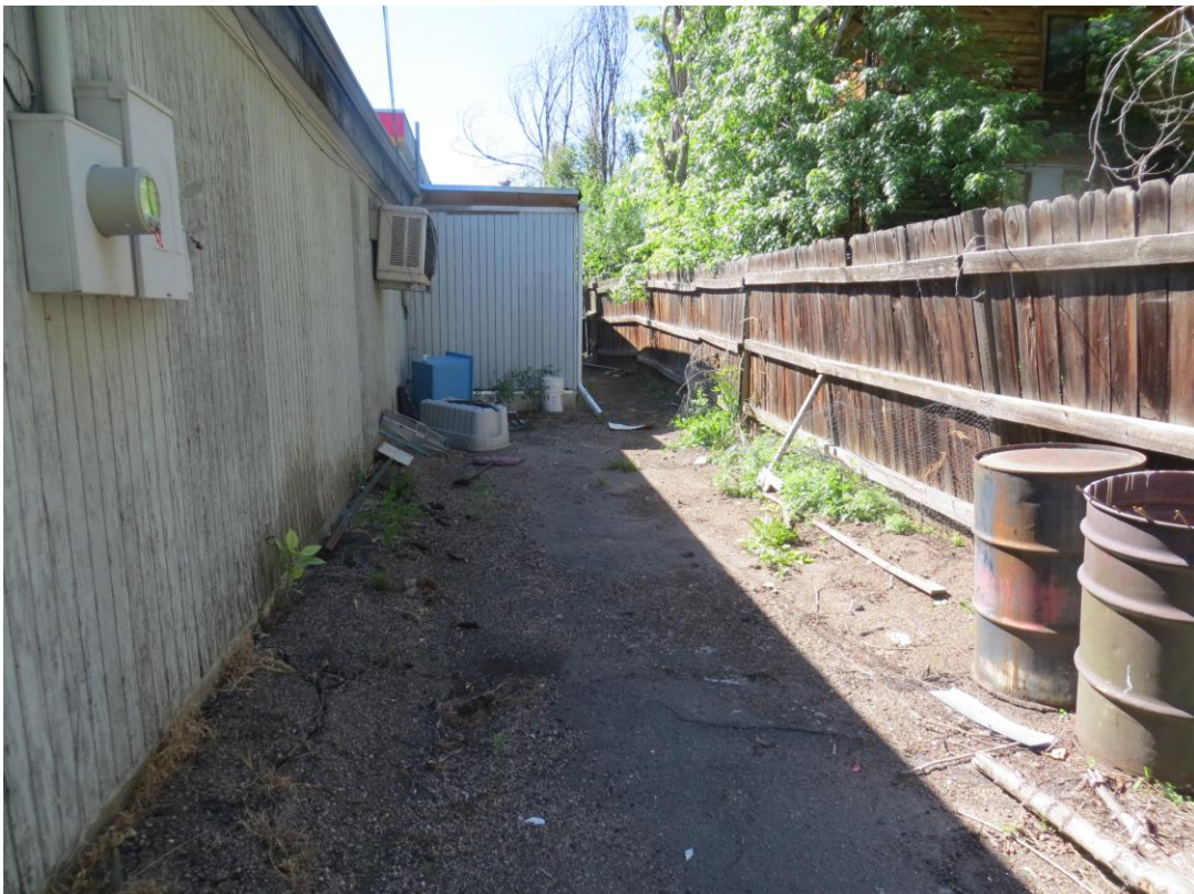
The back, or southwest side of the building.
