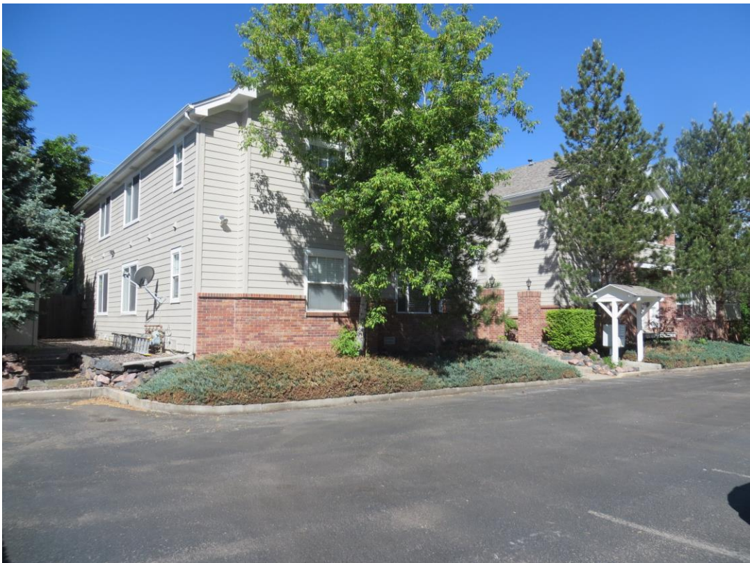
A multi-family residential property northwest of the subject property.
