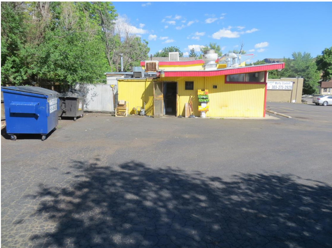
The southeast end of the building.
