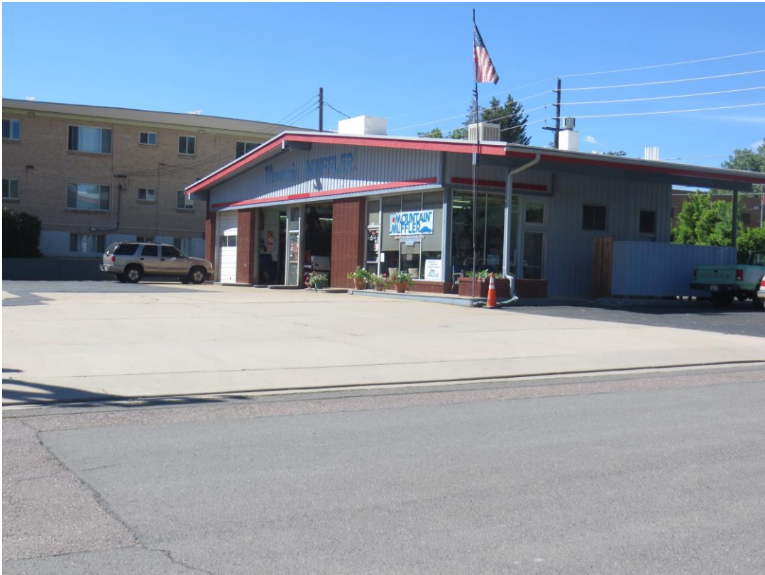
22 nd Street and a muffler shop are located southeast of the subject property.
