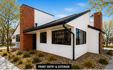
FRONT ENTRY & EXTERIOR
