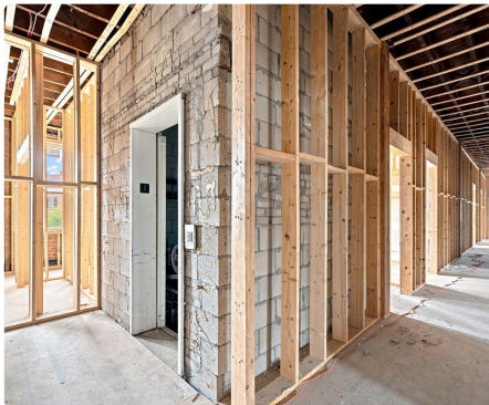
Framed corridor and existing elevator / block core
