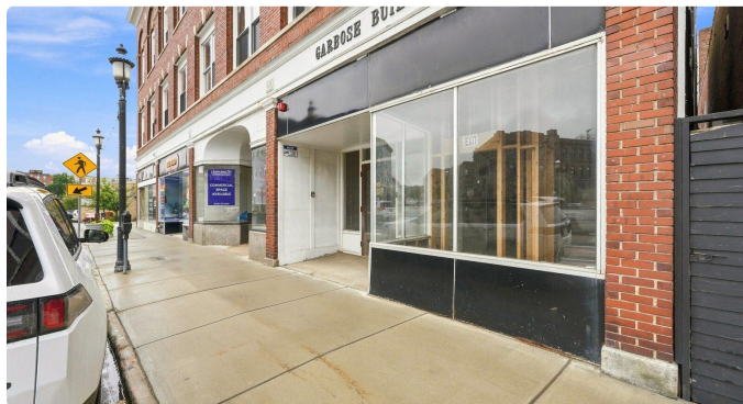
Garbose Building secondary elevation and available commercial frontage
