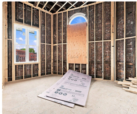
Corner unit framing showing original brick and arched window
