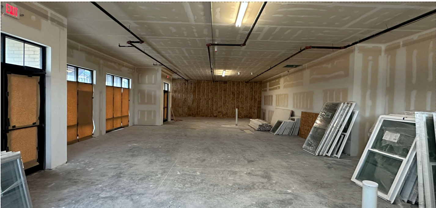
SUITE 002 — CURRENT SHELL CONDITION
