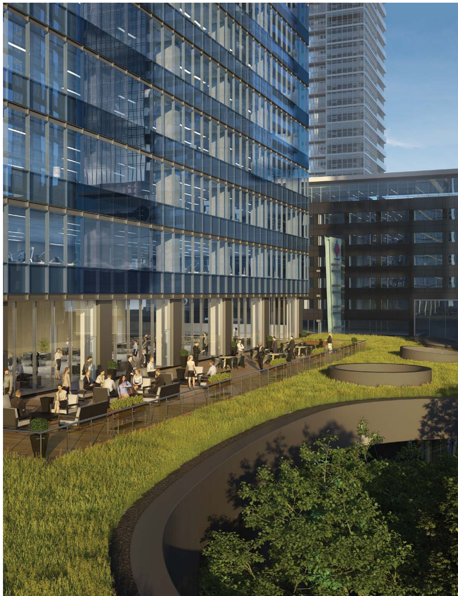
2nd floor tenant rooftop terrace
