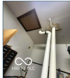
Mechanical room attic access
