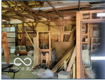
Interior of garage
