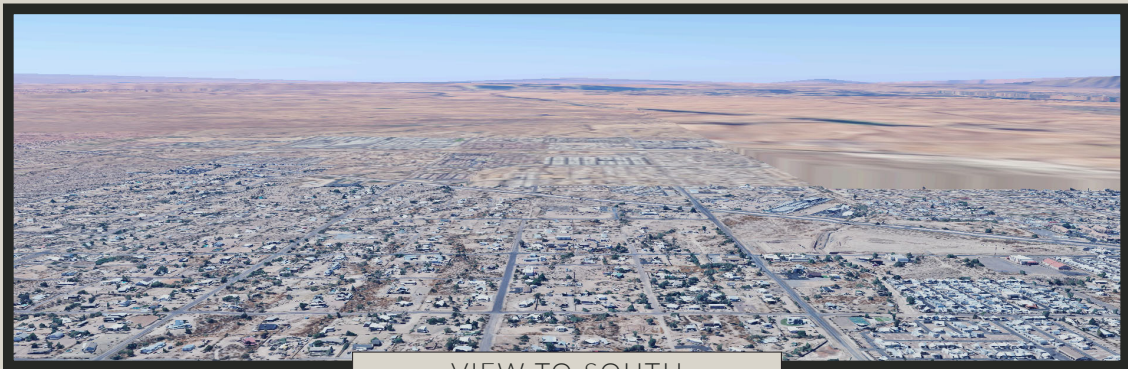
VIEW TO SOUTH
