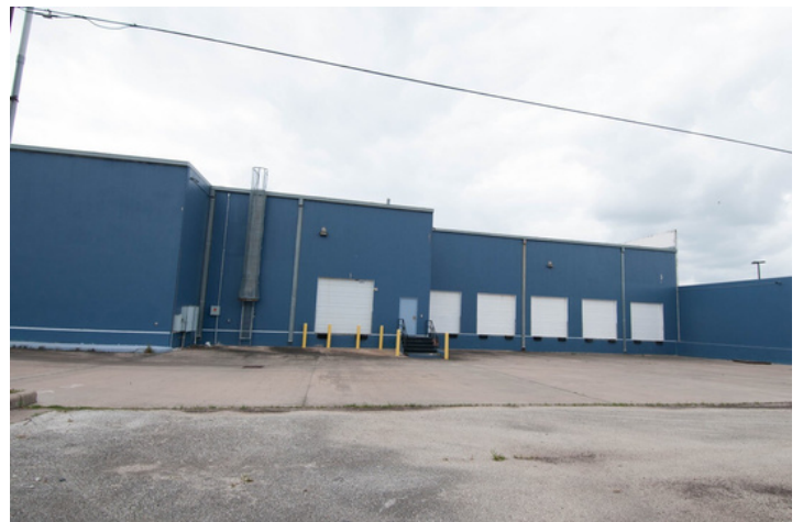
5 loading dock, 1 ground level, 2 customer pickup with ramps
