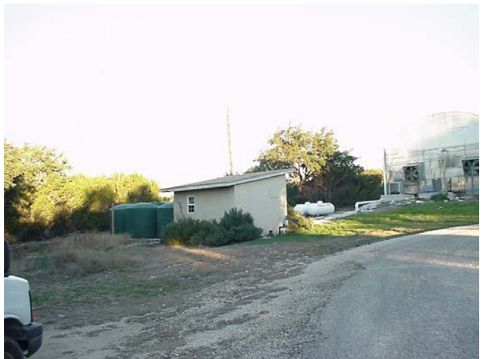
Shed located in front of greenhouses.
