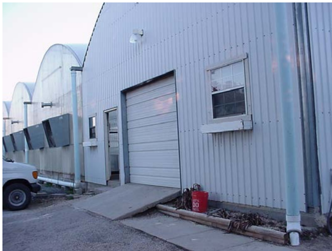
Overhead delivery door accessing the offices.
