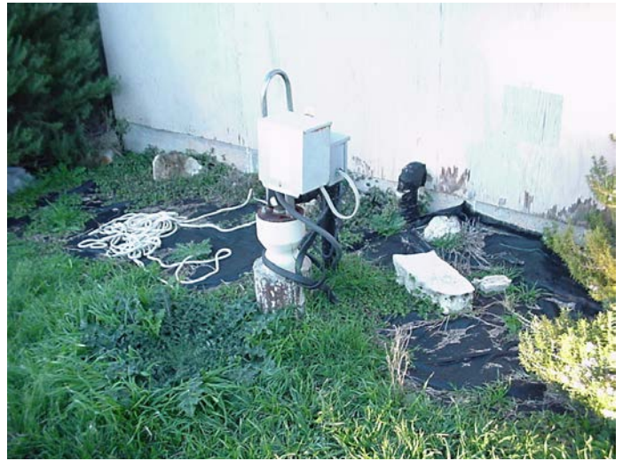
Water well located adjacent to the shed.
