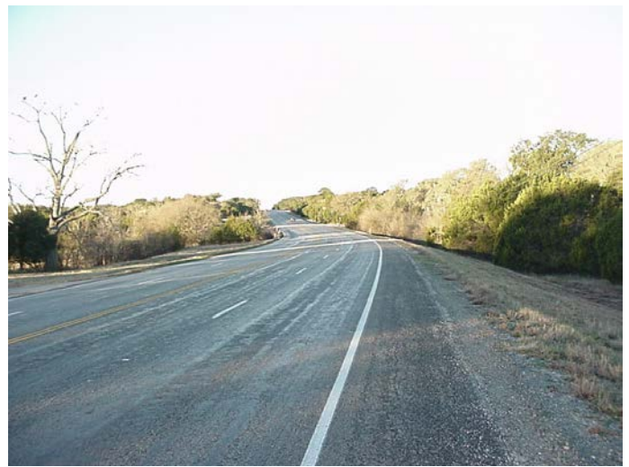
Viewing west along Highway 290.
