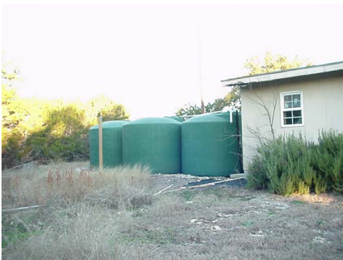
Plastic rainwater storage tanks located on the site.
