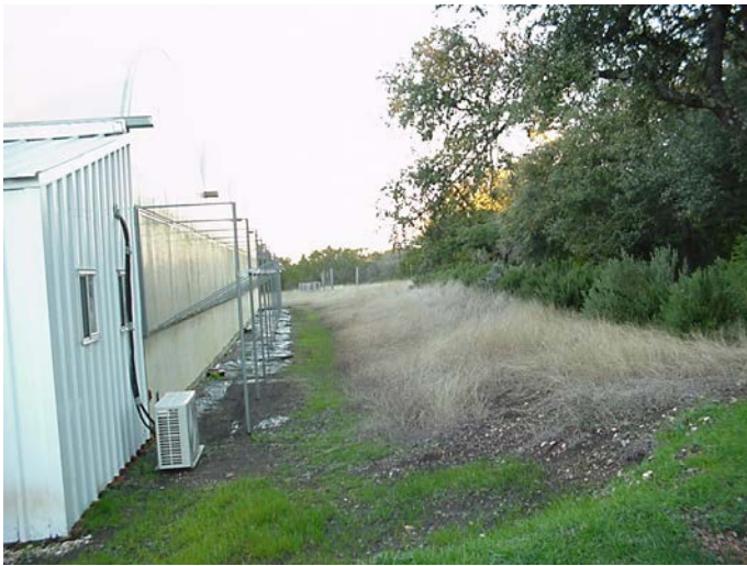
View behind (north side) the greenhouses.
