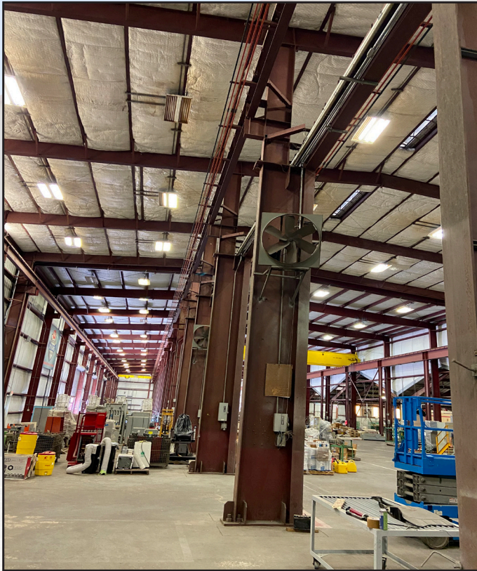
Interior of High Bay Fabrication/Manufacturing Shop
