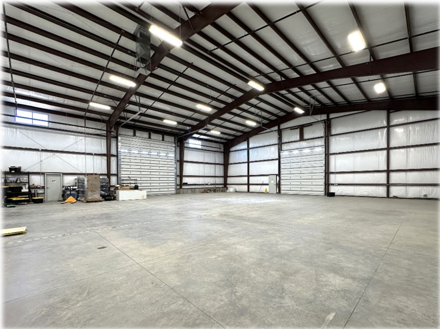
A-6 – South Side of Building A
