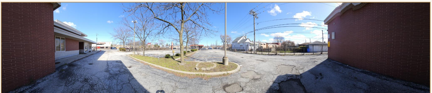
Main lot panorama (March 2024) — parking lot slated for full replacement; replacement proposal on file
