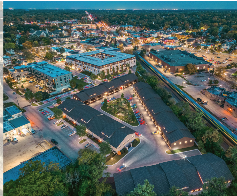
Currently Under Construction (Mylo Development)
