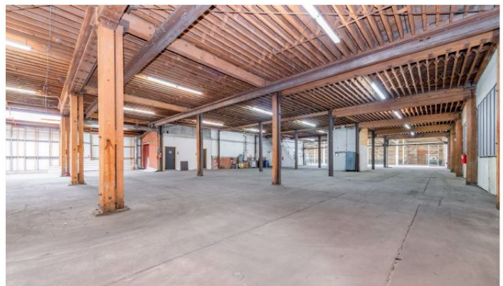
ORIGINAL 1918 WOOD-FRAME INTERIOR
