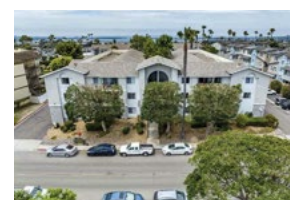
03 Bay Ridge Apartments
