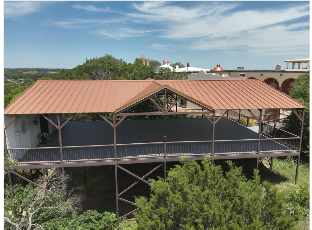
Pavillon side view
