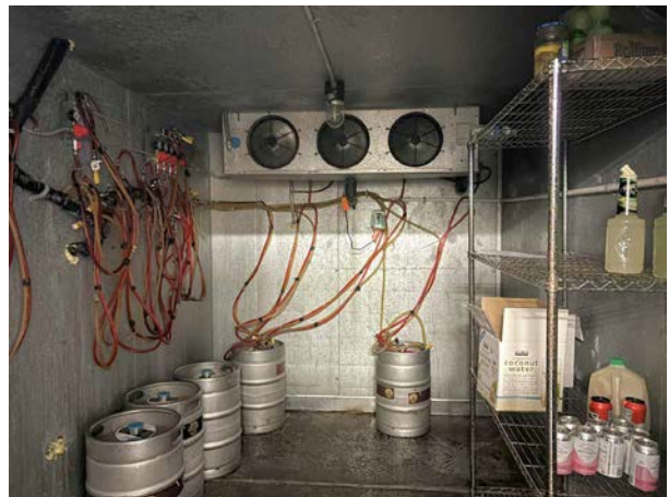
Lower Level - Walk-In Cooler
