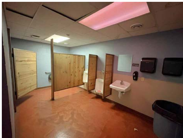
Lower Level - Restroom
