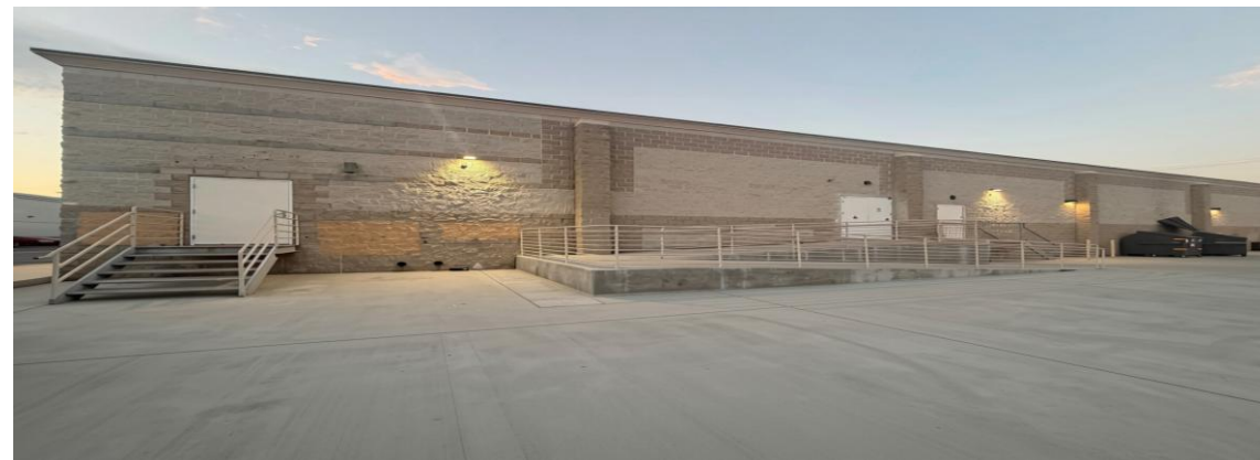
Rear ramp access, additional bay
