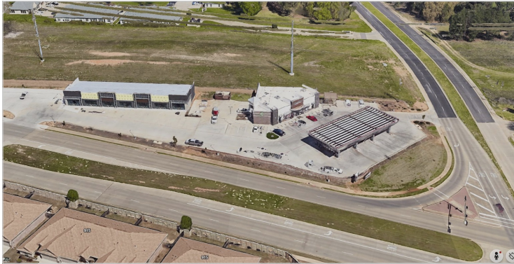
BIRD'S EYE AERIAL — SUBJECT PROPERTY & PHILLIPS 66 ADJACENT
