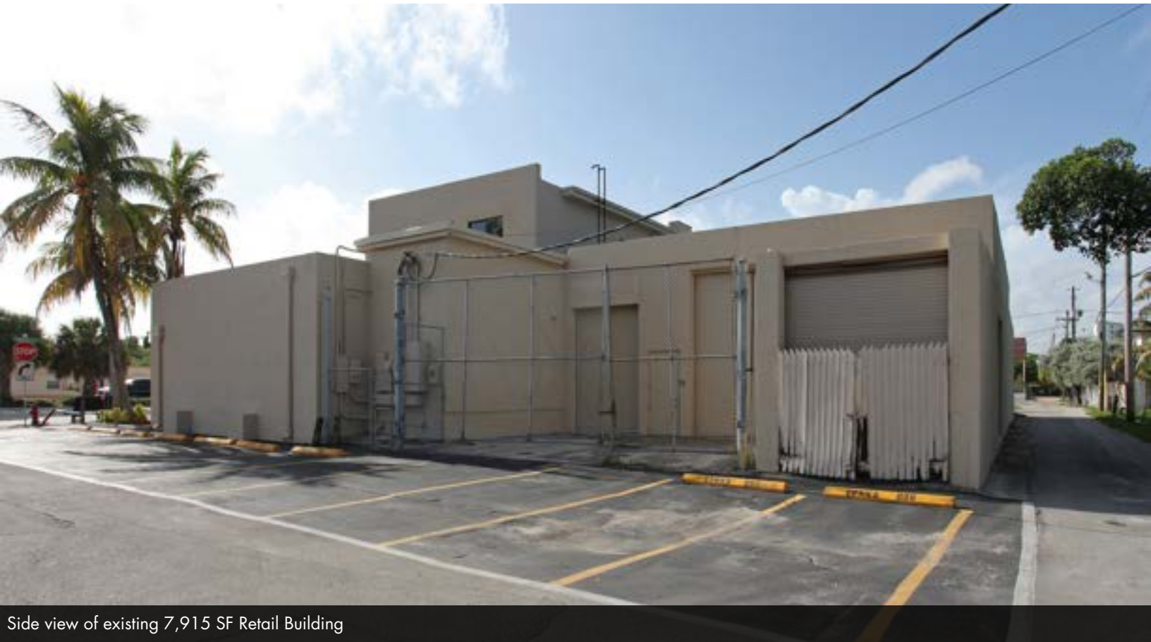
Existing 7,915 SF Retail Building
