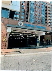
Parking garage behind the bldg.
