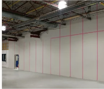
FIRE-TAPED DRYWALL — WALLS & CEILING
