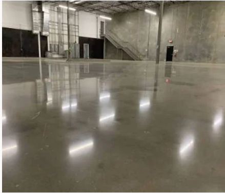
SEALED CONCRETE FLOOR
