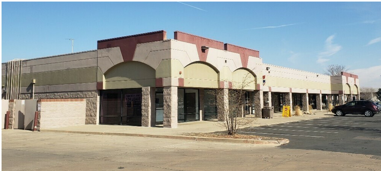
14311 E. 4th Ave. Exterior
