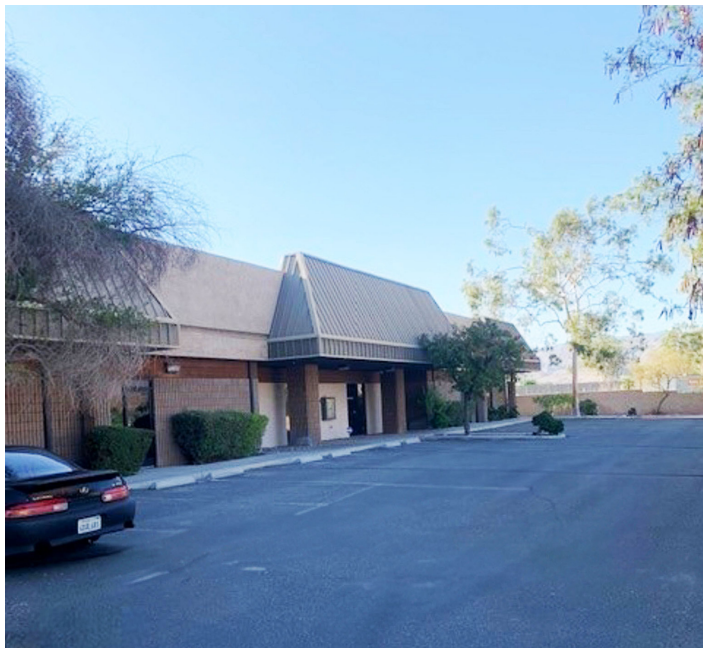
Building Rear Parking
