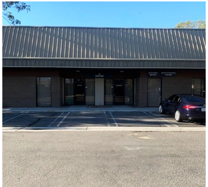
Building Rear Parking
