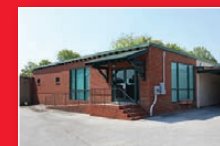
Building D 2,466 Sf
