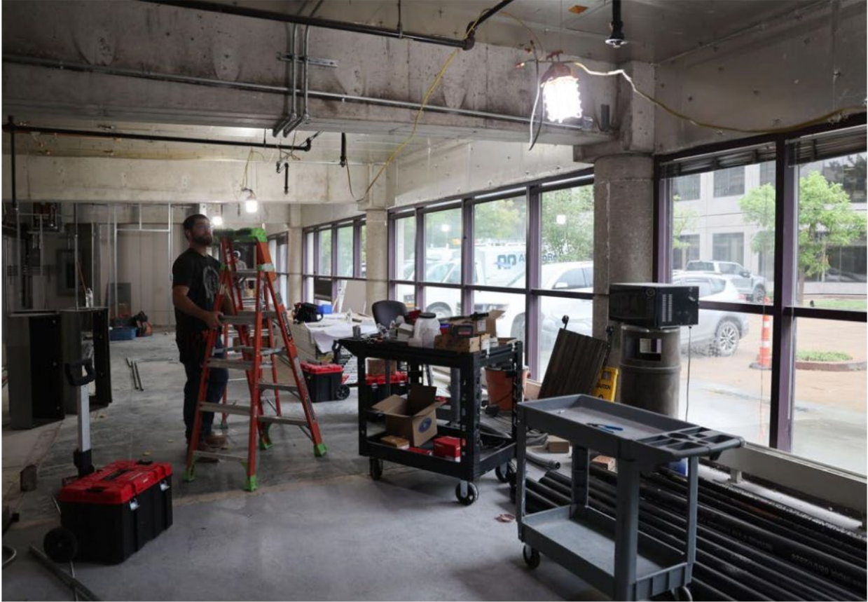
Warren Place is undergoing $20 million in renovations. Stephen Pingry, Tulsa World
