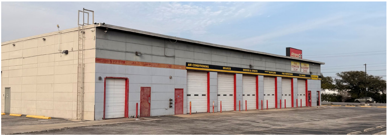
■ 6-bay auto repair facility
