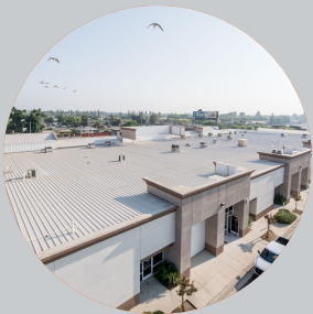
WELL MAINTAINED ROOF
