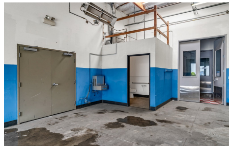
Interior corner — restroom & office access
