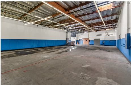
Warehouse — alternate view
