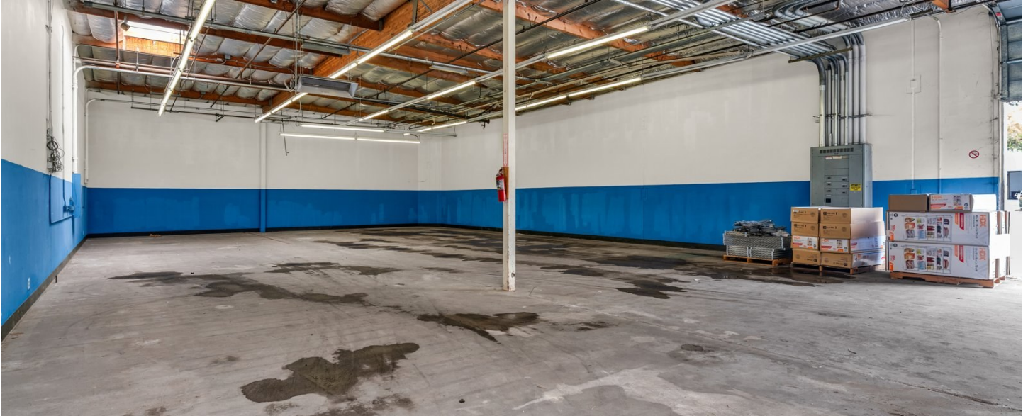
Open warehouse interior — exposed wood ceiling, ±3,240 SF clear span
