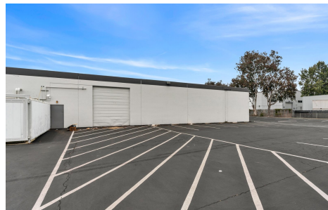
Side parking & access
