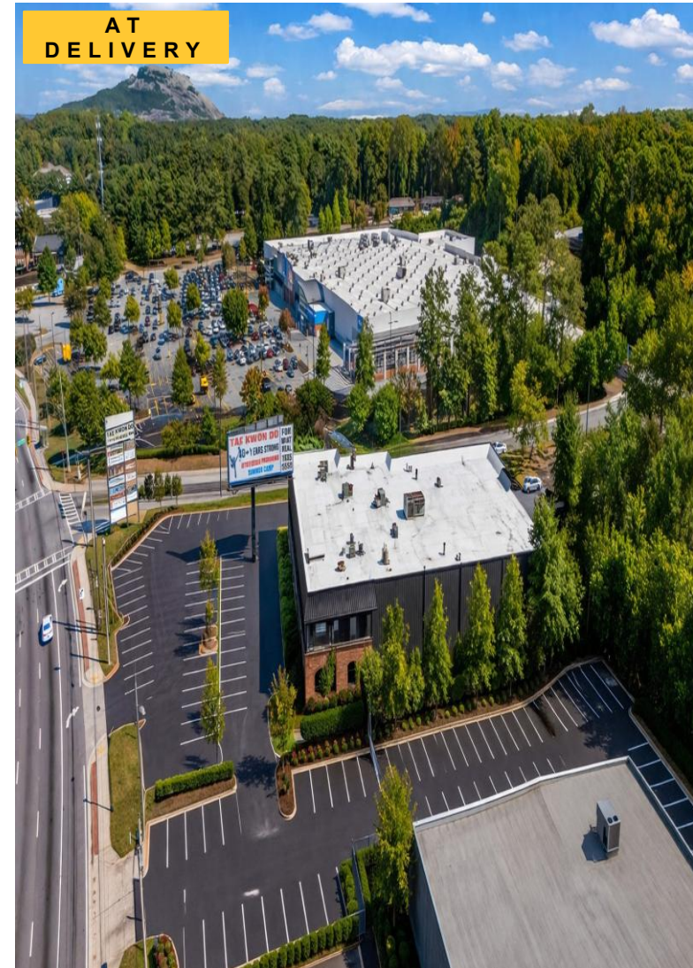
Aerial · subject corridor · Stone Mountain backdrop
