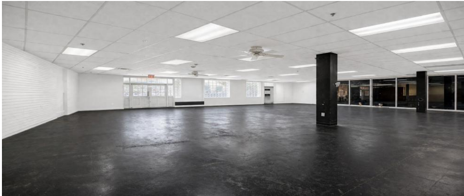
Photo 01 · existing fitness/dance bay (black floor, ceilings)
