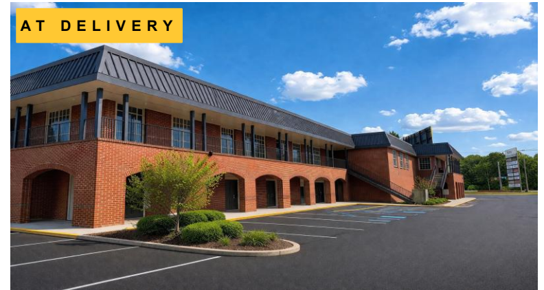
Front parking · pylon view from corridor
