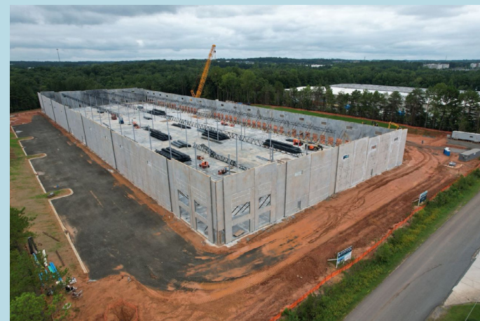
Construction Update: Walls and Steel Going Up
