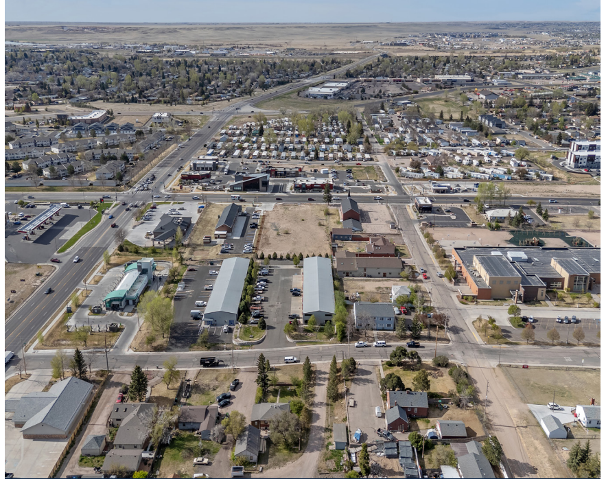
CENTRAL CHEYENNE LOCATION WITH INTERSTATE ACCESS
