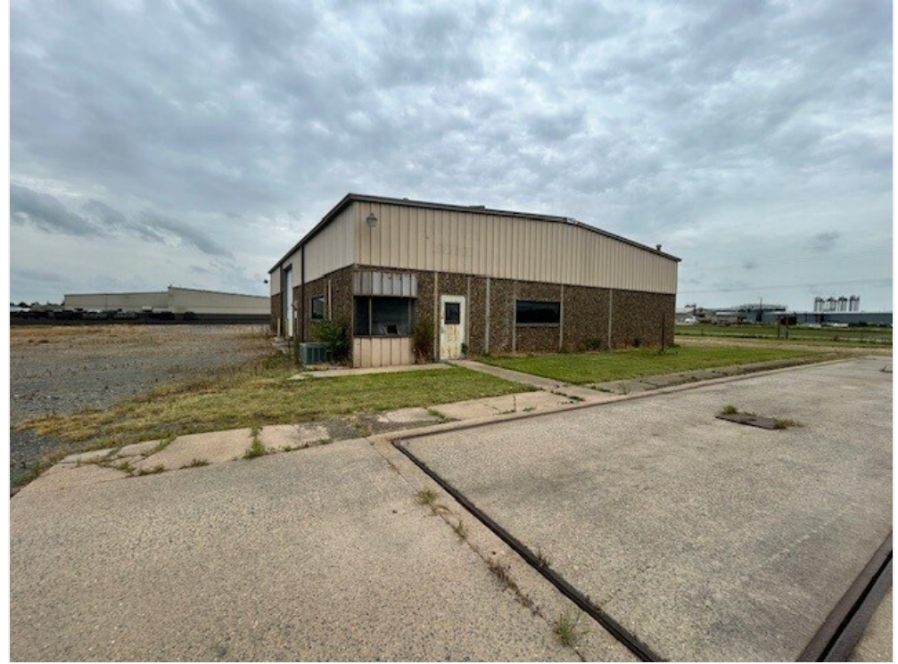
Office inside warehouse/Scale
