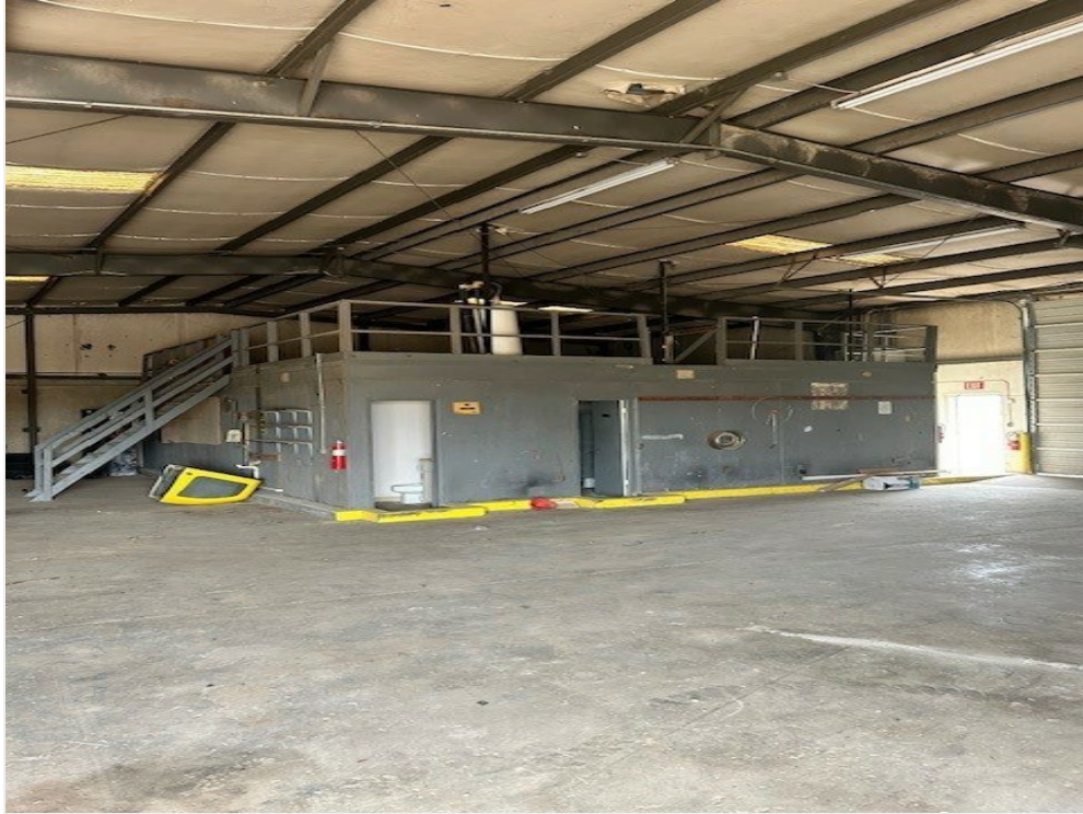
Office inside warehouse/Scale
