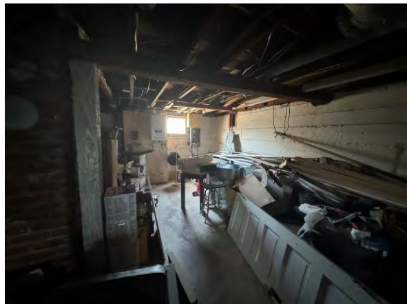
Subject interior – Basement/lower level
