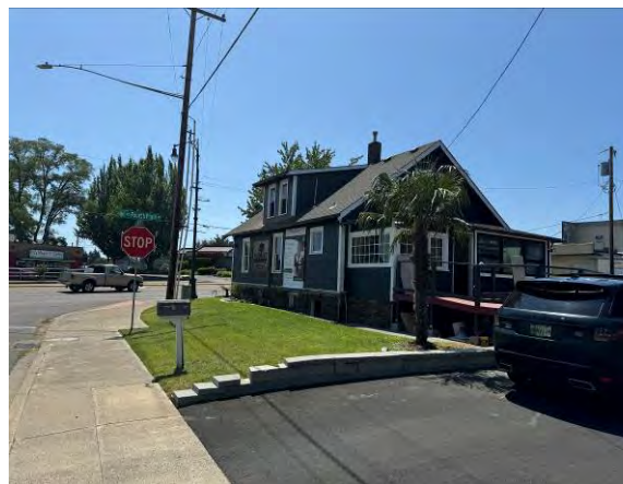
Subject property looking southwest
