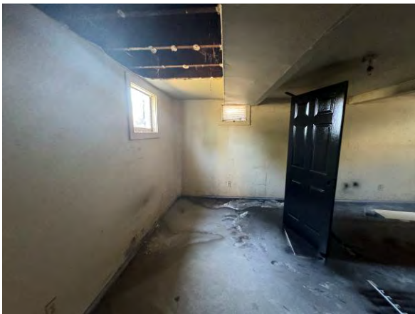
Subject interior – Basement/lower level
