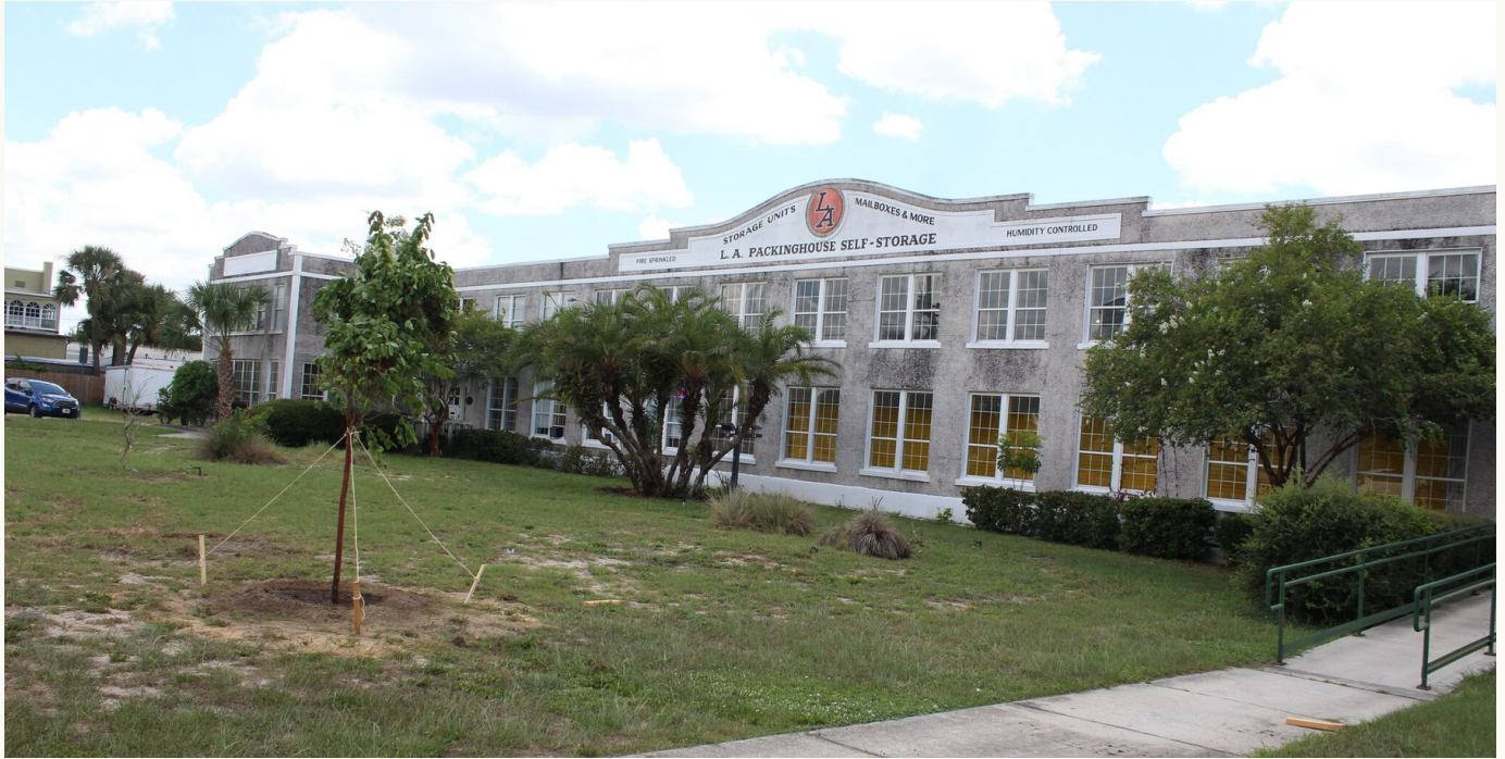
TWO-STORY MASONRY FRONT BUILDING — W HAINES BLVD ELEVATION
