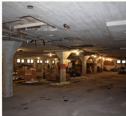
BASEMENT — MUSHROOM COLUMNS
