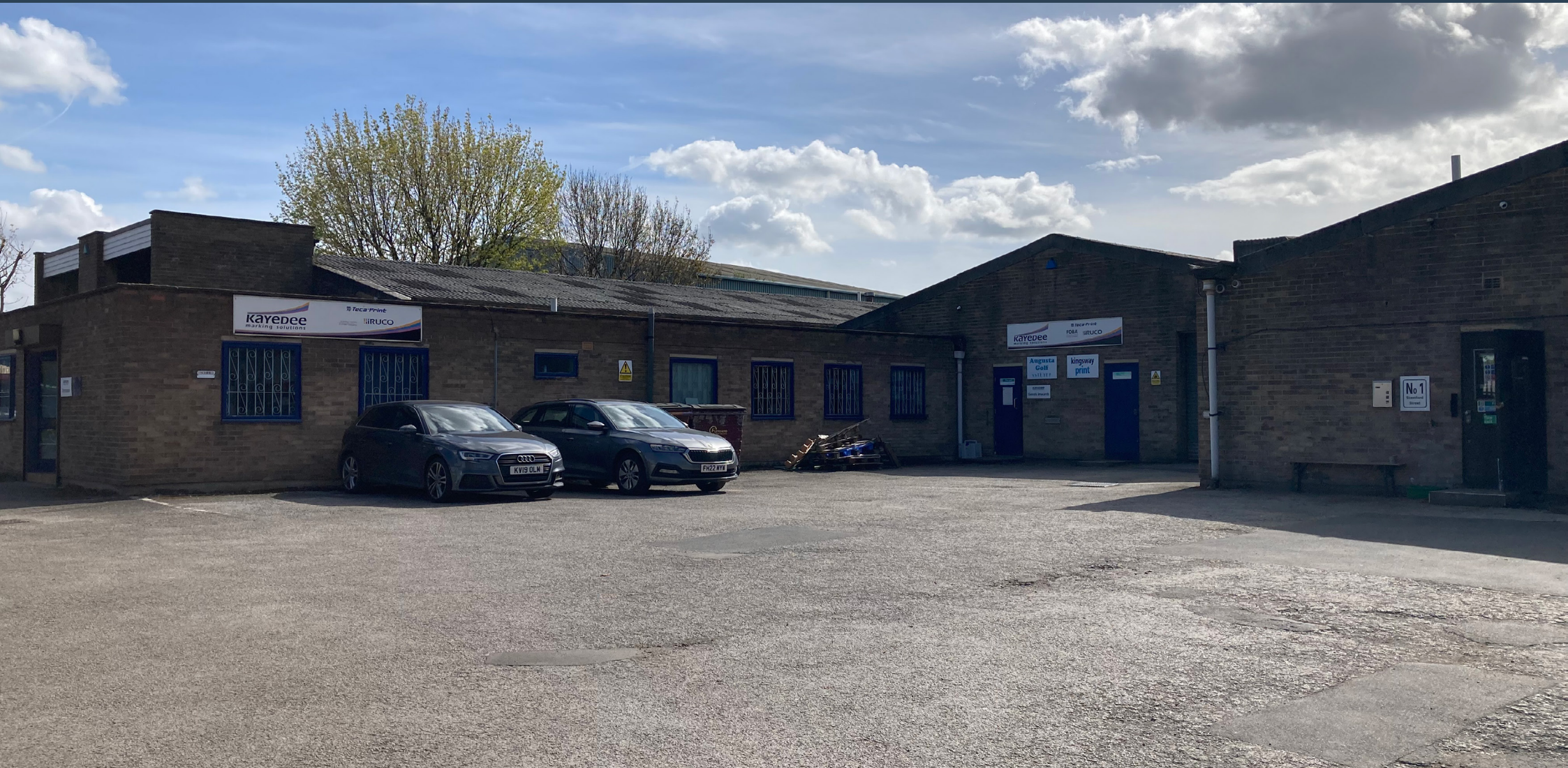
Kayedee Premises, Stamford Street, Newhall Road Trading Estate Sheffield, S9 2TX
