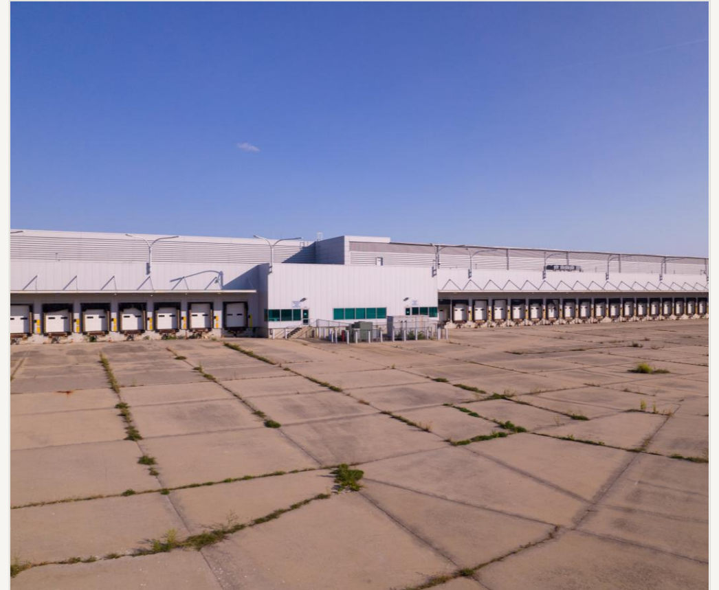
— Dock line and high-bay storage within the distribution building.
