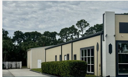
Office Building Exterior
