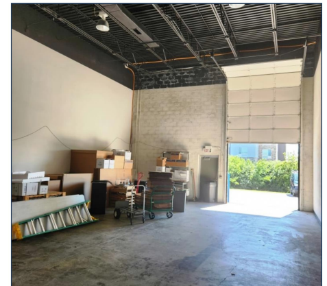
WAREHOUSE - DRIVE-IN DOOR
