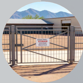
±3,300 SF OUTSIDE STORAGE
