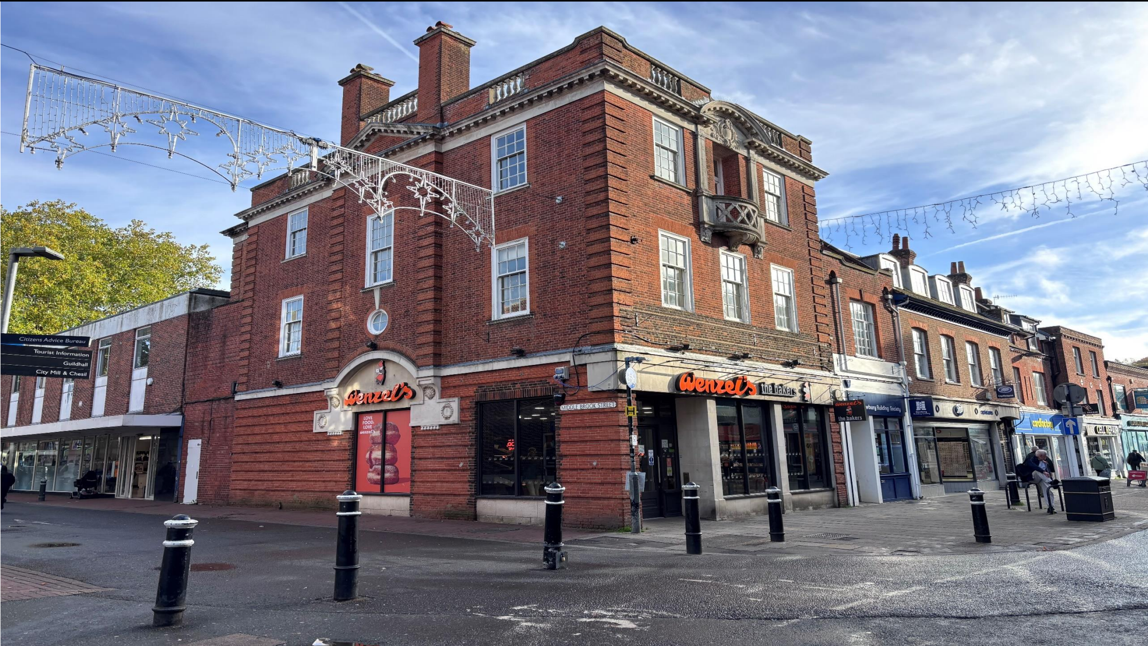
Ground Floor, 141-142 High Street, Winchester, Hampshire SO23 9AY
