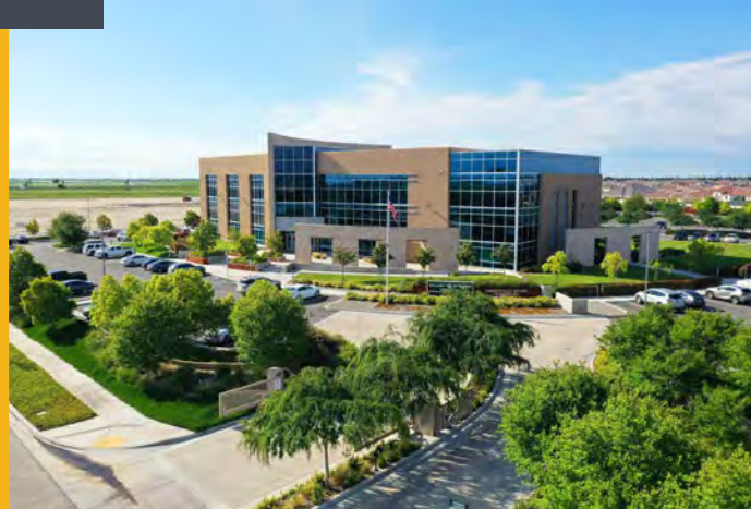
Valley Strong Credit Union 60,000 SF Headquarters
