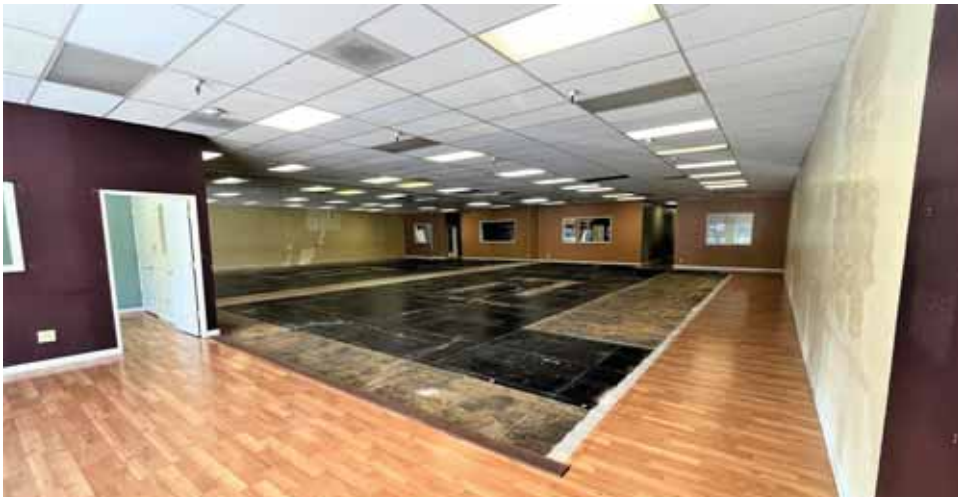
6940 Interior - Former Martial Arts Studio
