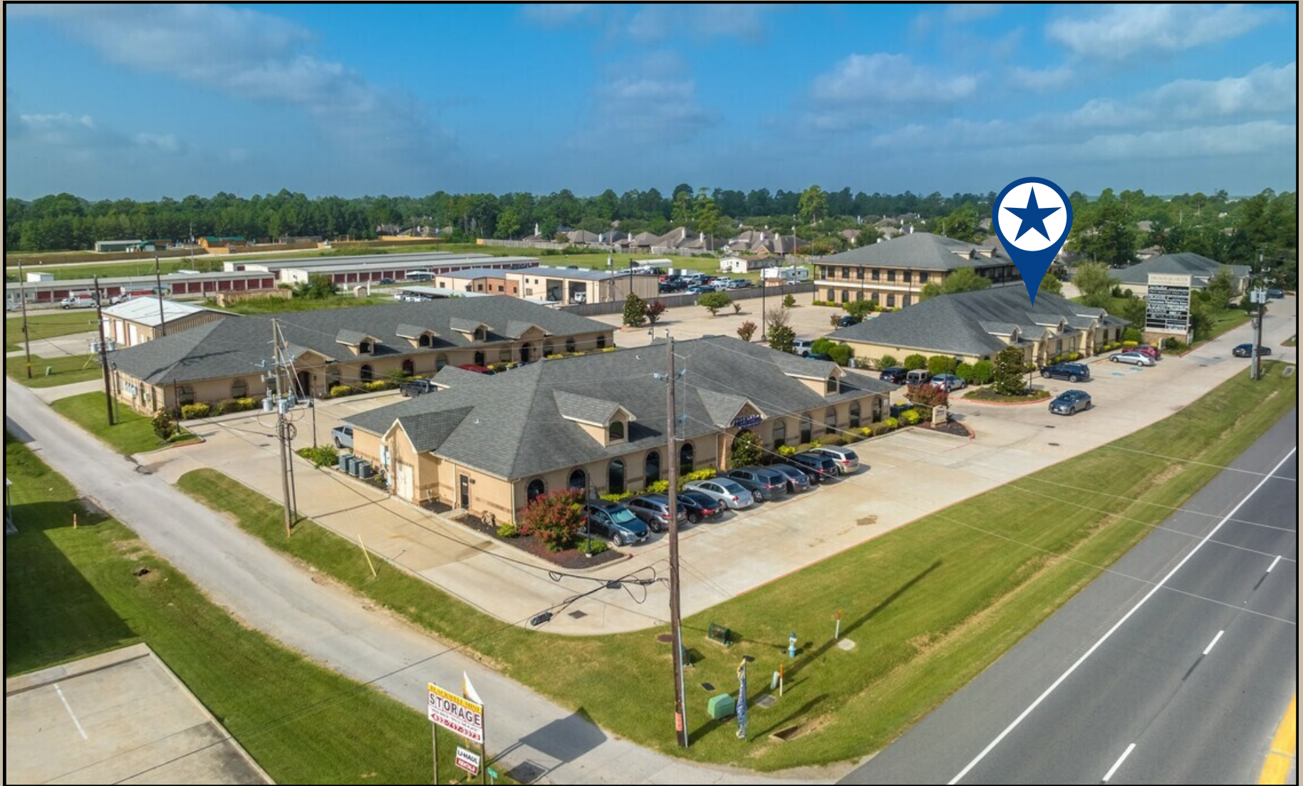
Corner Aerial View
