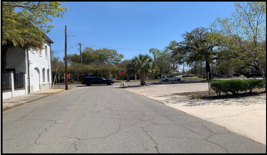
Easterly View Along East York Street With 129 East Broad Street Located In The Right Background
