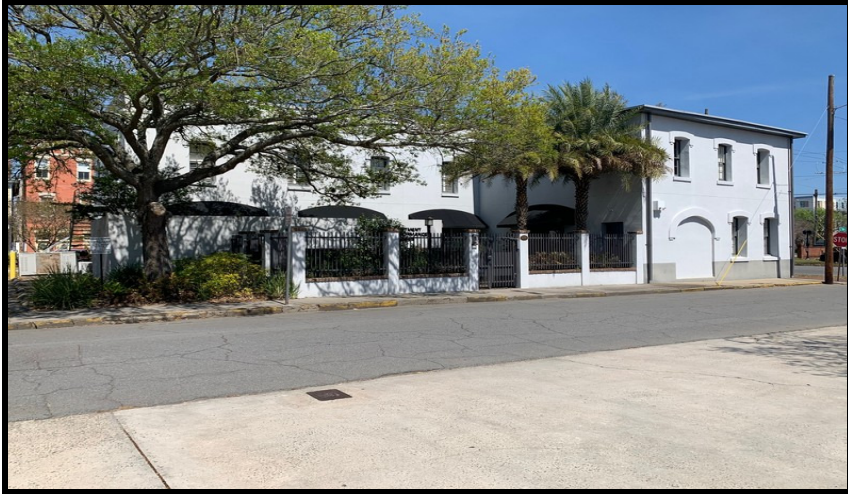
View Of The Southern (Front) Elevation Of 570 East York Street
