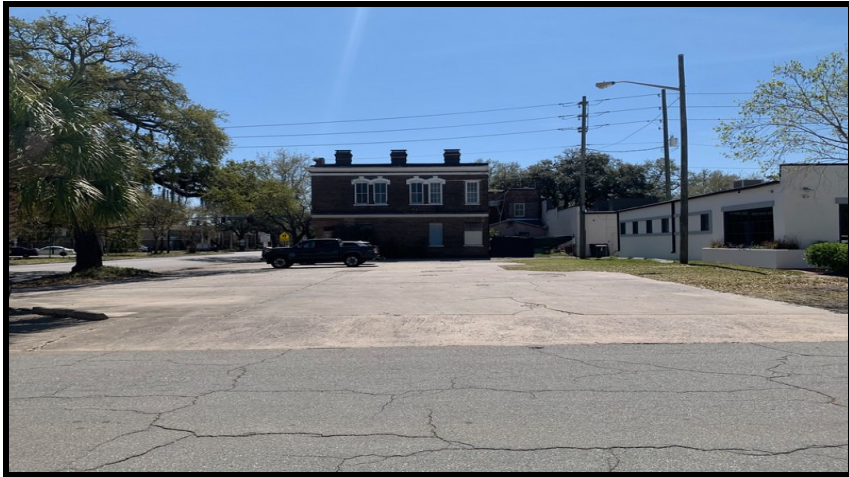
Southerly View Of 129 East Broad Street From East York Street
