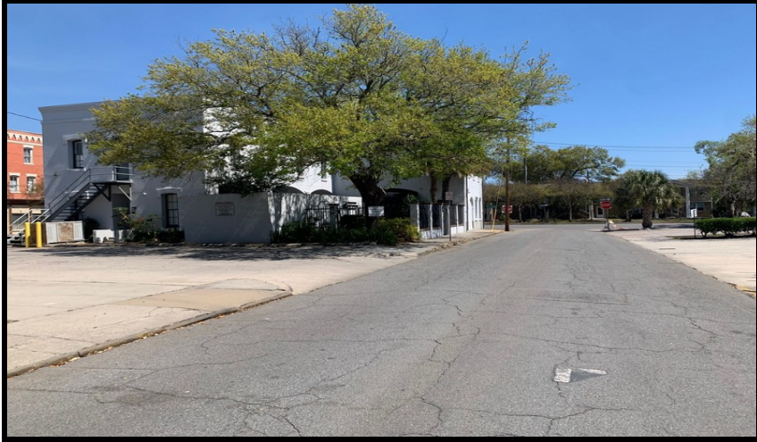
Easterly View Along East York Street 570 East York Street Is Located At Left Background
