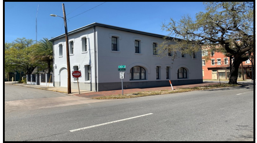
Views Of The Eastern And Partial Southern Elevations Of 570 East York Street
