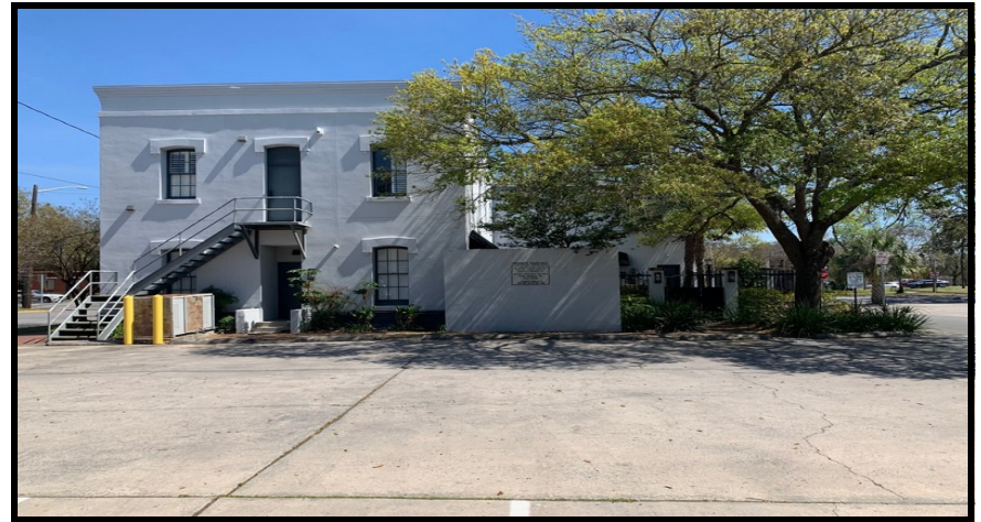
View Of The Western Elevation Of 570 East York Street
