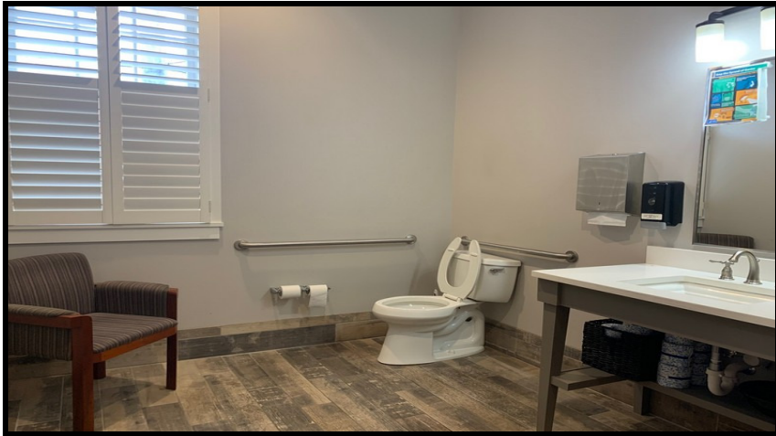
View Of A Typical Second Floor Restroom
