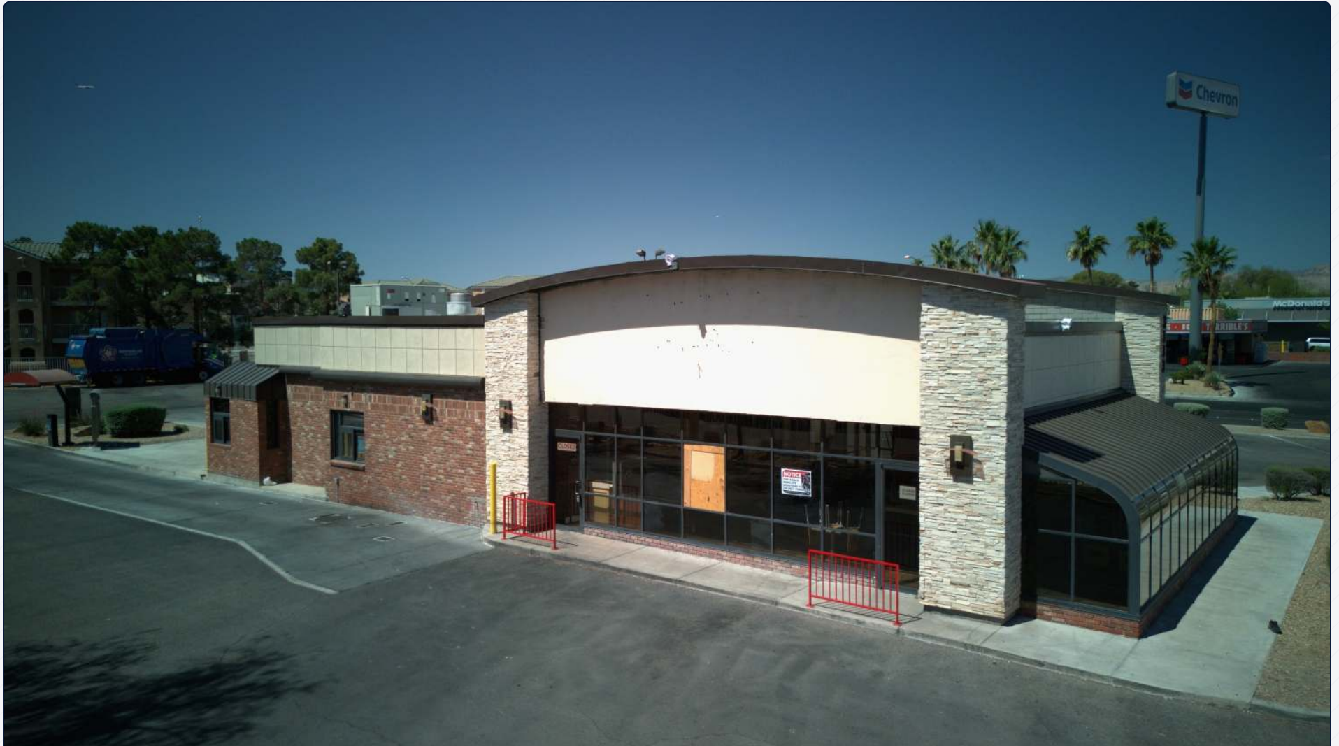
SUBJECT BUILDING ELEVATION Drone photography — brick & stone façade with drive-through-improved pad
